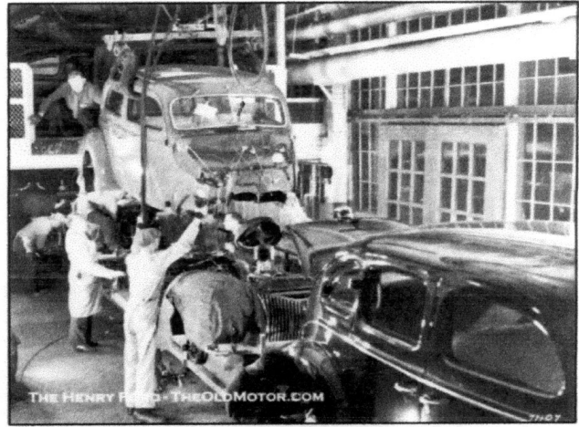
A Deluxe 1939 Ford Tudor body is lowered onto its chassis. This car might have been a special order. The page affixed to the windshield was probably the "build sheet" and it looks like the car has a radio antenna installed on the roof between the windshield wipers.
