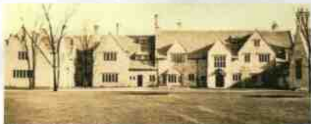
Edsel and Eleanor's Grosse Pointe home was completed in 1929.
