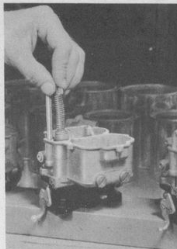
Figure 91—Removing Accelerating Pump
